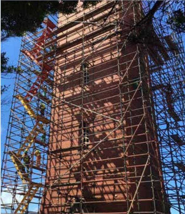
*Scaffolding being erected up the 52meter high Campanile in preparation for phase 1 of the restoration process.*
