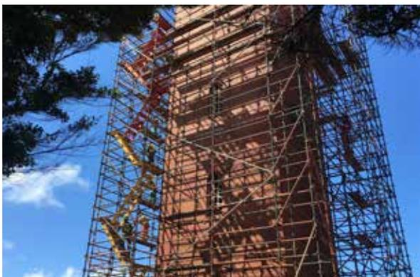
*Scaffolding being erected around the 52m high Campanile in preparation for phase 1 of the restoration process.*
