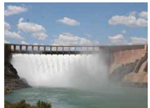
*The 80 metre high Gariep dam that holds back the mighty Orange River, with its 914 meter long doubleway road running on top of the structure.*
